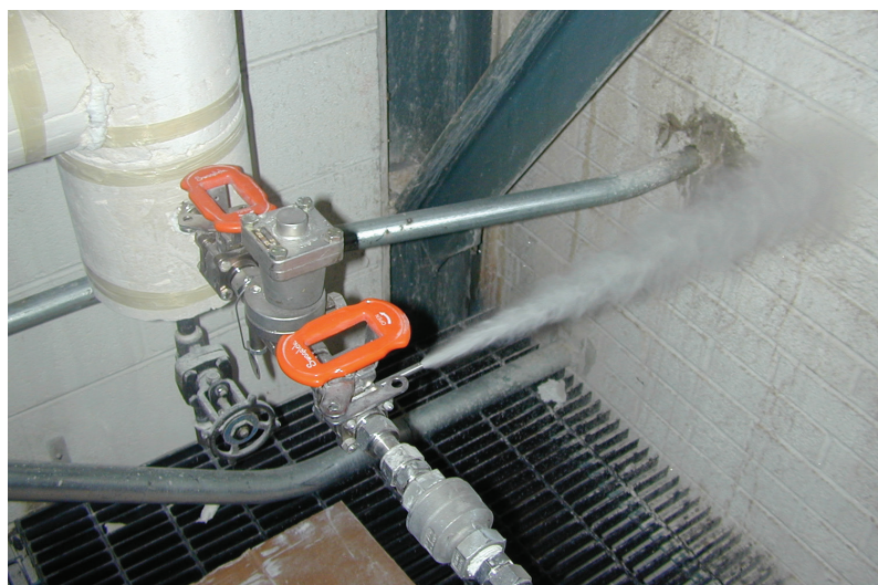
Figure 2: Steam Trap – Discharging Flash
