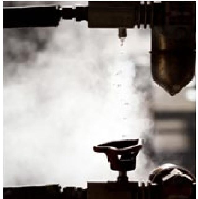
*Figure 3: Visual testing for steam traps*
