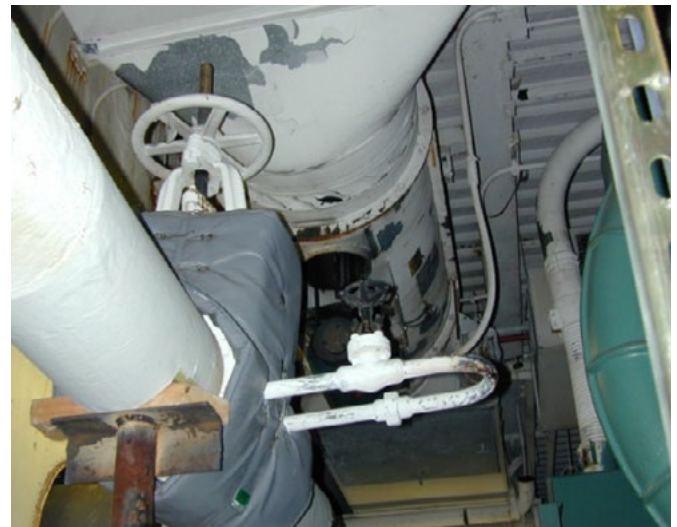
Figure 3: Isolation Valve with a Warm-Up Loop
