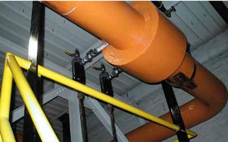
*Figure 3: Flow metering with Condensate Chambers*
